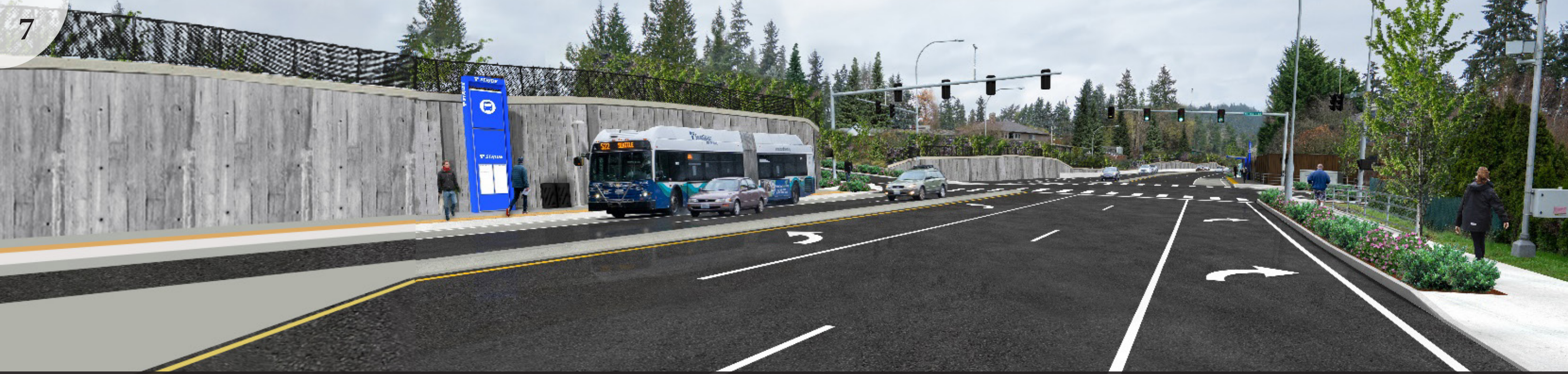
SR 522 NE 145 BRT Wall and Black Chain Link Fence Do Not Provide Noise Mitigation
