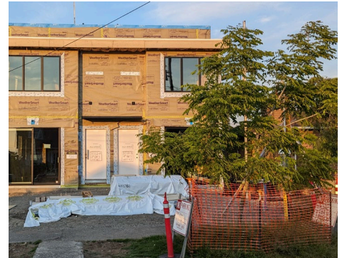
Example of a new middle housing development that is protecting existing trees. Source: MAKERS
