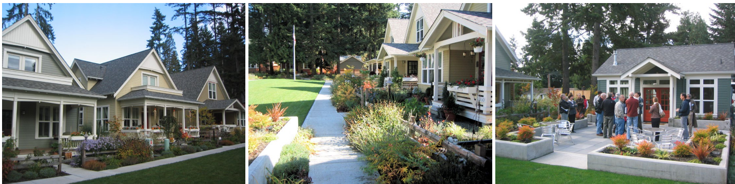
Danielson Grove Cottages in Kirkland. Note the mix of private (landscaped areas in front of the cottages) and common (lawn area plus the patio) open spaces and community building example (right image). Source: MAKERS.
